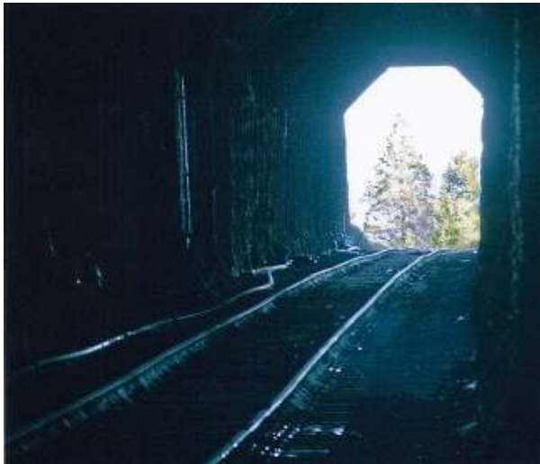
#56 – We walked back through the 0.8-mile-long tunnel a second time to look back across the summit hump, plainly visible here. (Like most tunnels, this one is not level, a deliberate feature which allows it to drain water.)
